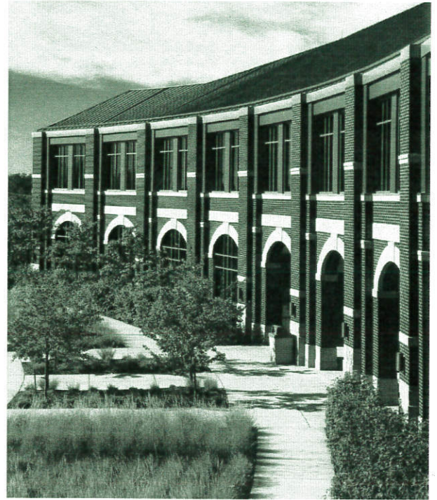
Metro Patrol Division Station—7601 Prospect Ave
