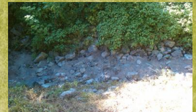
Many of the larger rocks had been washed from the West side of 77 th street over to the East side. Work was done to remove the rocks, shore up the banks and put concrete in to keep future storms from washing more rocks away.
